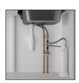
Check for leaks and turn 4 the cold water supply back on and flush/run for 30 seconds.
