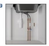
Install the filter to the cold water filter diverter valve, making sure that the direction of flow matches the arrows on the filter head.
